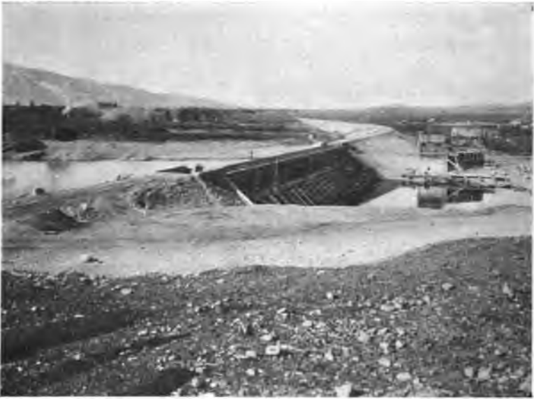
FIG. 98.—Jackson Lake Dam, Downstream Face, Wyoming.
